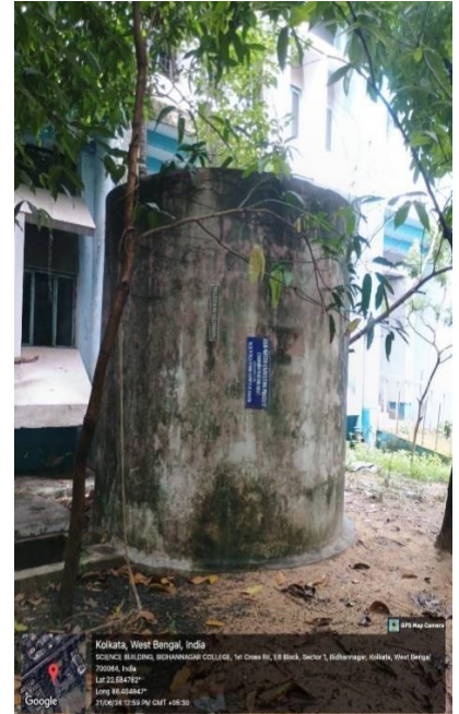
2. Rain water harvesting Unit
