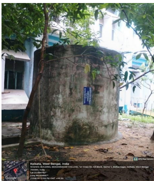
Rain water harvesting unit of Bidhannagar College
